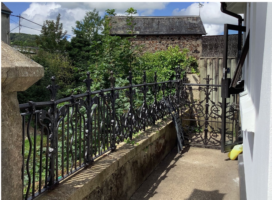
Traditional decorative ironwork
